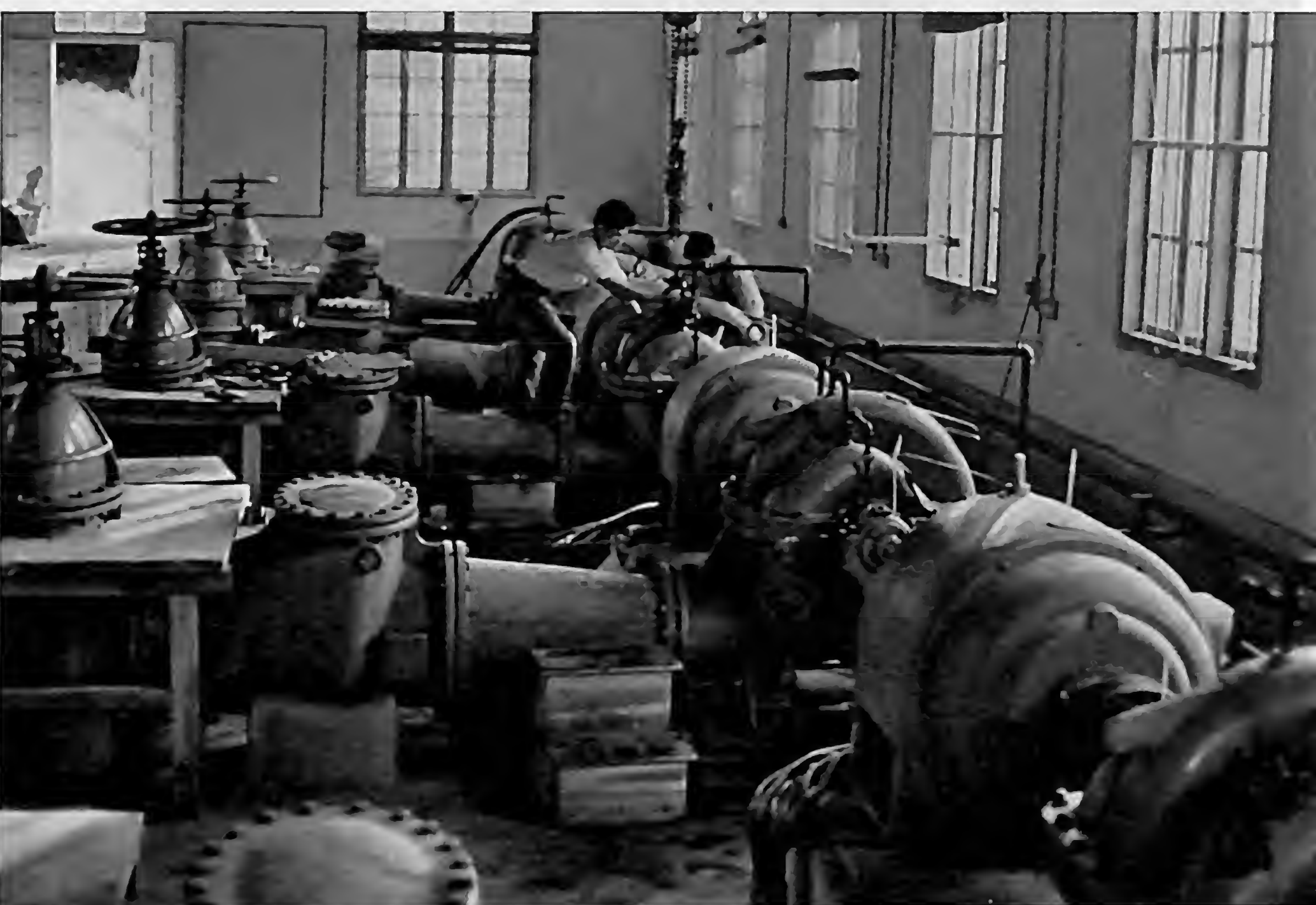
The county-run machinery plant produces power equipment in large quantities for use in water conservancy.
